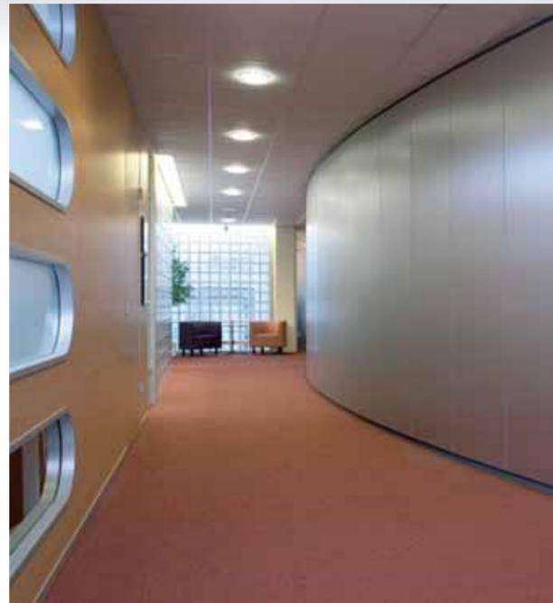
system is created with double plaster board panels, which increase the sound insulation value. The two systems can be combined without requiring adaptations. More and more architects and interior designers opt for Interfinish partition systems, which combine well thought-out aesthetics with practical advantages such as straightforward installation and the ease with which they can be rearranged.
